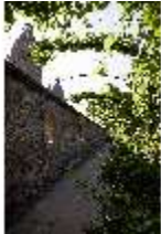
AschPomp.V, Laubengang (sog. Kapuzinergang), DI015031, BSV-
