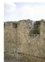
SaZwe.I, Burgmauer (Detail), DI008226, BSV-
