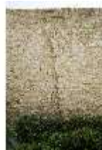
SaZwe.I, Wehrmauer (Detail), DI008225, BSV-
