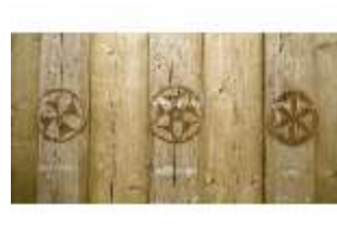
Pr.II, Holzdecke, Detail, R.2, DI001220, BSV
