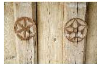
Pr.II, Holzdecke, Detail, R.2, DI001221, BSV
