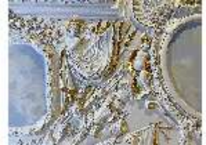
CoE.II, Riesensaal (Detail Stuck), R. 9, DI020888, BSV-
