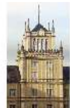
CoE.I, Hauptfassade, Turm, DI009201, BSV-
