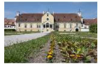
SAS.I, Ostfassade, DI014465, BSV
