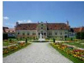
SAS.I, Ostfassade, DI009737, BSV
