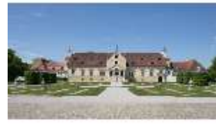
SAS.I, Ostfassade, DI014464, BSV
