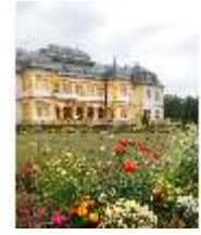
Vh.I, Westfassade, DI014645, BSV-
