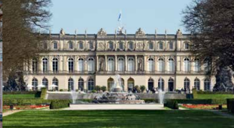
Herrenchiemsee Palace (New Palace)
