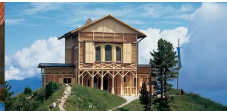
King's House on Schachen
