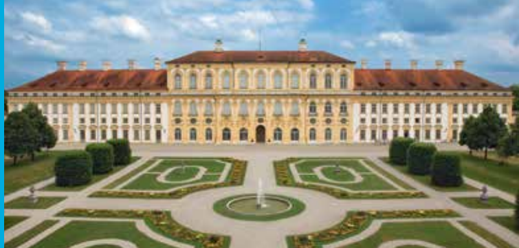
Schleissheim New Palace
